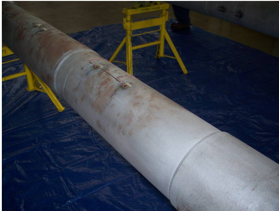
Figure 46 – Sandblasted surface of pipe prior to installed work
