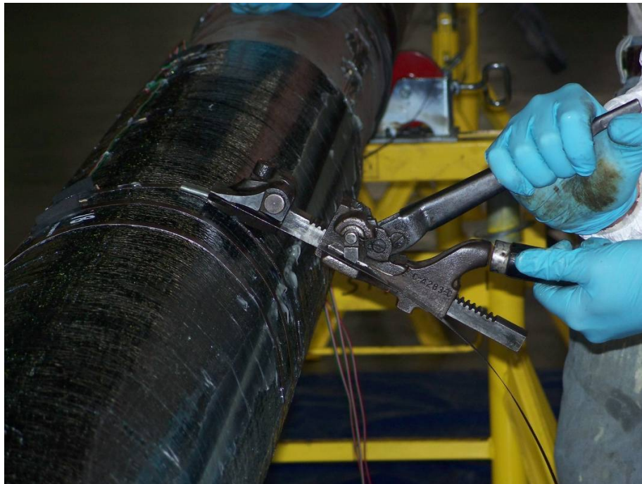
Figure 53 – Installing steel banding clamps on the outside of the half shells
