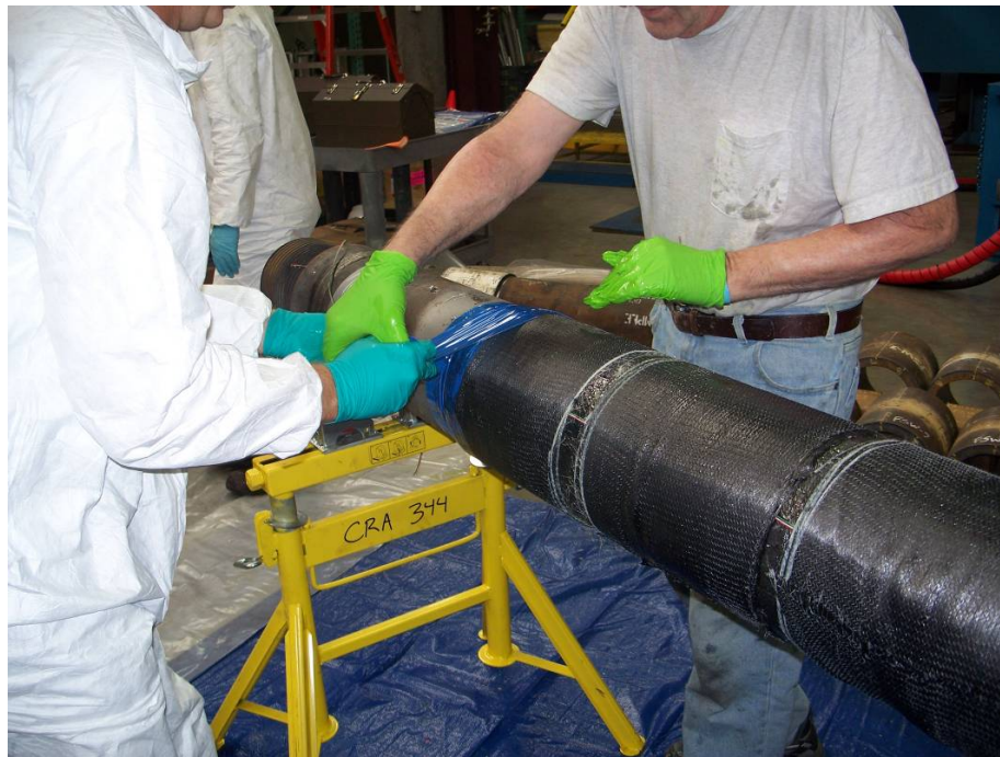
Figure 54 – Installation of the outer hoop carbon and stricker wrap material
