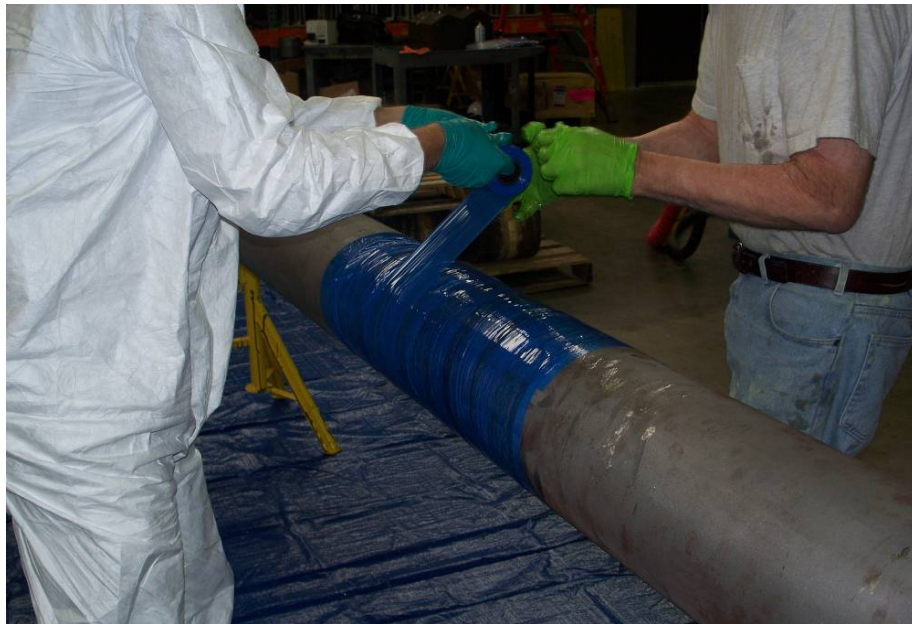
Figure 49 – Installing stricker wrap material around the outside of the repair
