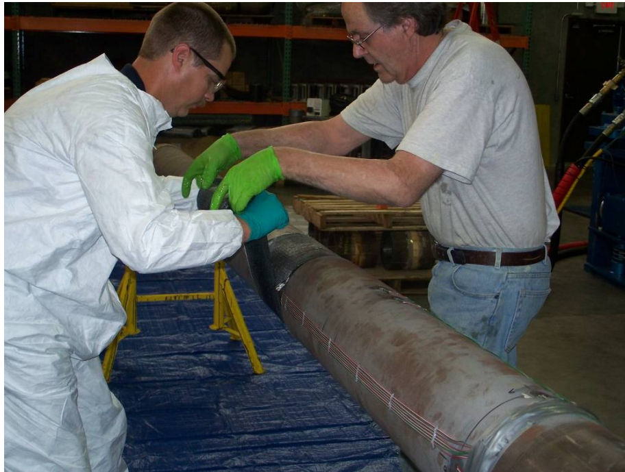
Figure 48 – Installing the hoop wrapped inner carbon layers
